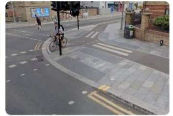
Figure 4.84 Example of mini zebra crossing of cycle track and pedestrian landing area (Image: Google Street View)
