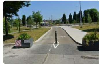
Figure 2.2 Example of a seamless transition from a quiet street to a cycle track, Eden Park, Dublin
