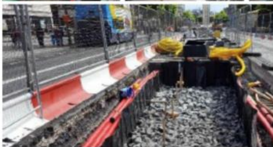
Figure 25 Stockholm tree pit system under construction in O'Connell Street
