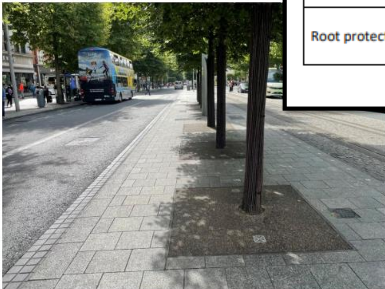
Figure 26 Completed scheme for the Stockholm tree pit system in O'Connell Street Dublin
